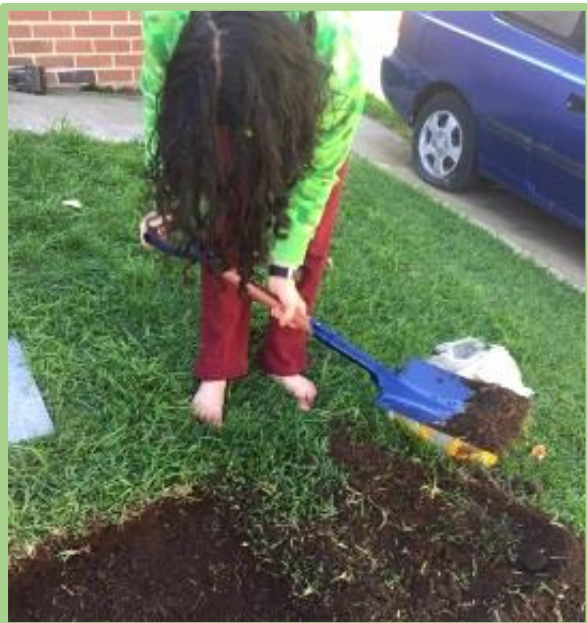
Tommy laying pavers
